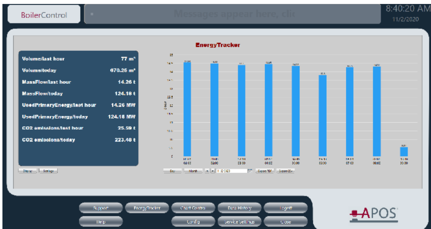
Screenshot BoilerControl EnergyTracker
