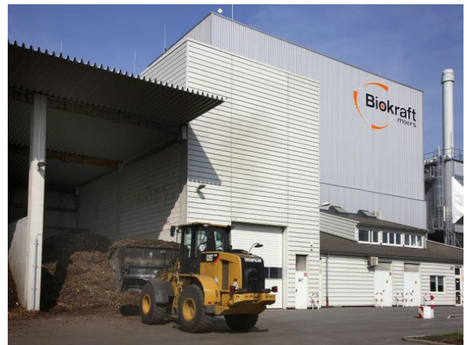
Biomass combined heat and power plant Moers
