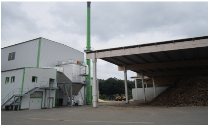
Biomass CHP Hosenfeld
